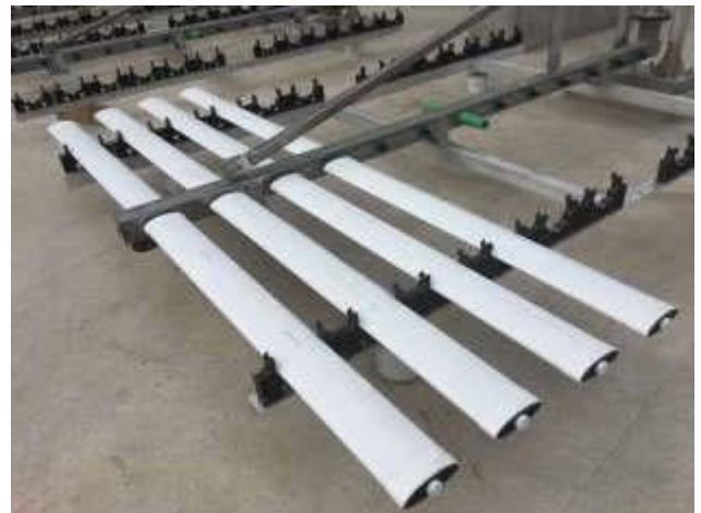
Component 2: Aeration diffusers
