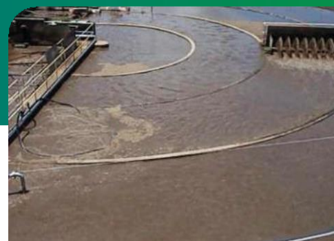
Activated Sludge Systems
