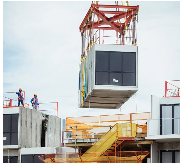
04 LIFTING AND ERECTION
