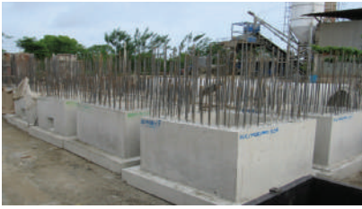
Washout Valve Chambers
