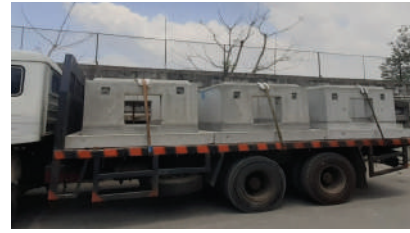
Air Valve Chambers
