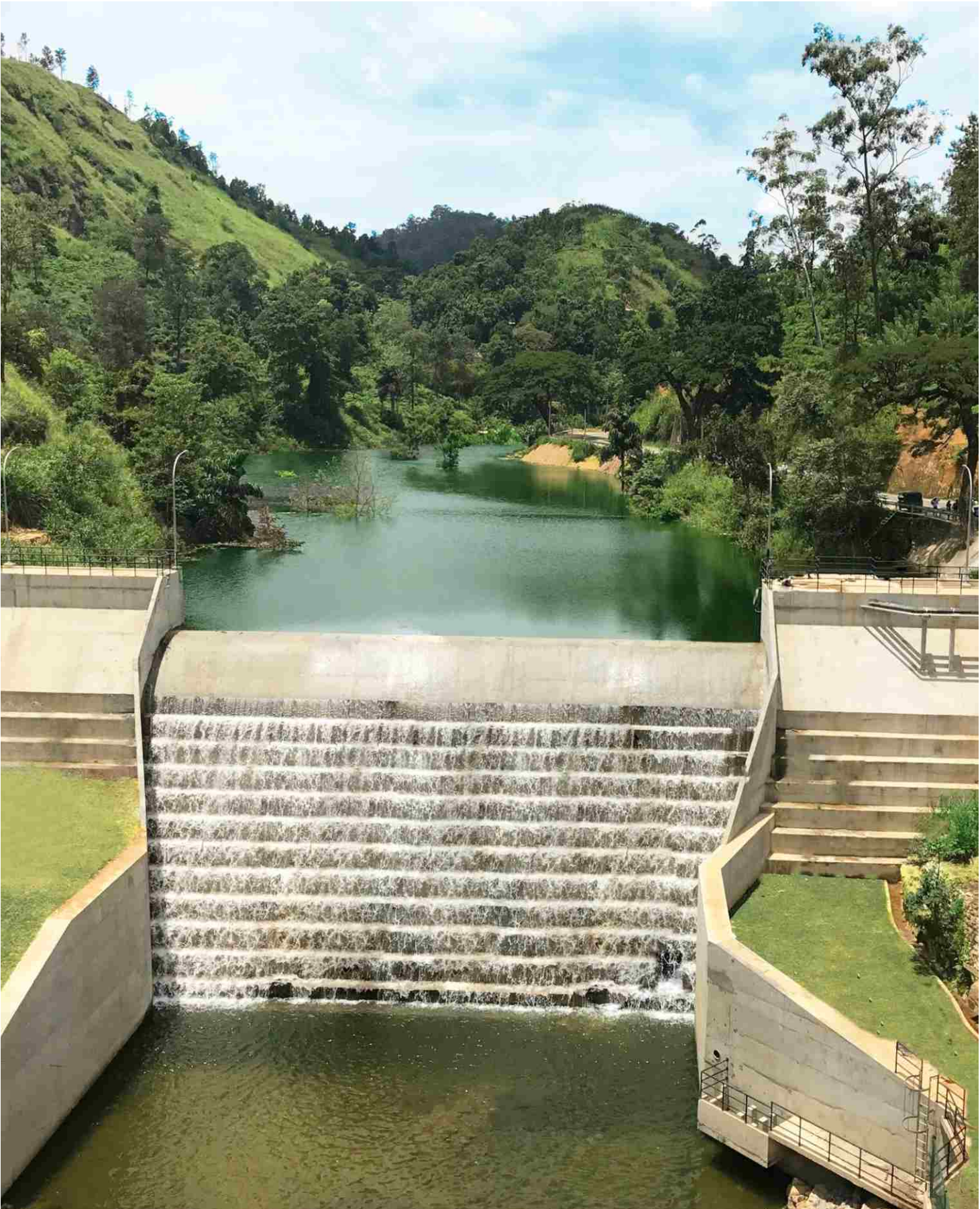
Water Supply Project - Hali Ela
