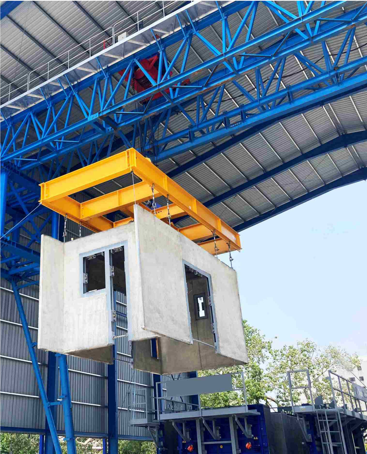
Prefabricated Prefinished Volumetric Construction (PPVC)
